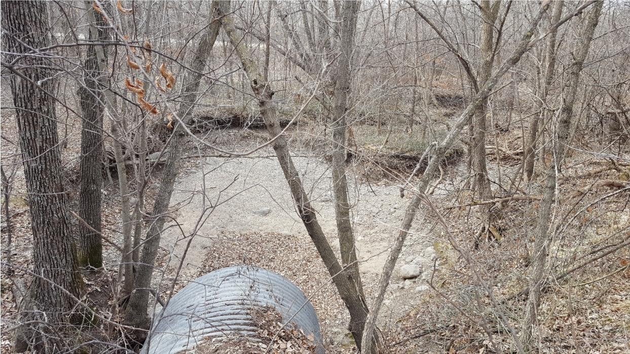
Recent, unvegetated ditch maintenance activity and insufficient buffer left some ditch channels susceptible to erosion and sedimentation.
