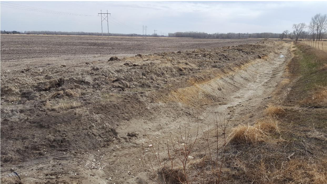
Excessive wind erosion and substantial deposition of wind-blown sediment within ditches was a common occurrence throughout the western portion of the Clearwater River Watershed in the spring of 2021.
